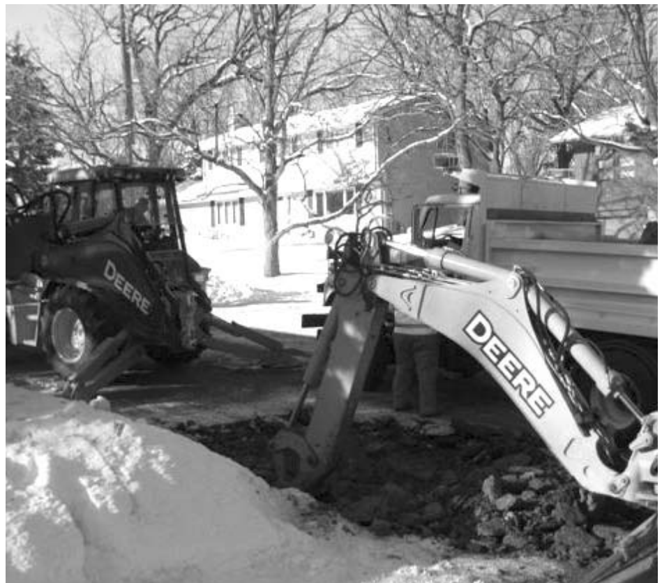
Typical water main repair, winter of 2008.
