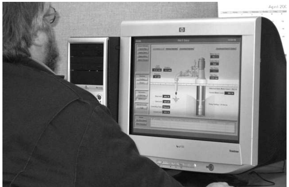
Kris Fluegel, Treatment Plant Operator, monitors the City's water system utilizing the SCADA system at the Water Treatment Plant on 5th Street.
